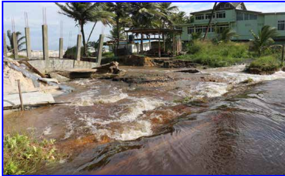
Flood waters undermine a foundation at a beach house in Manzanilla
